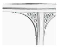
Image shows gallows brackets fitted to gutter channel and post.
